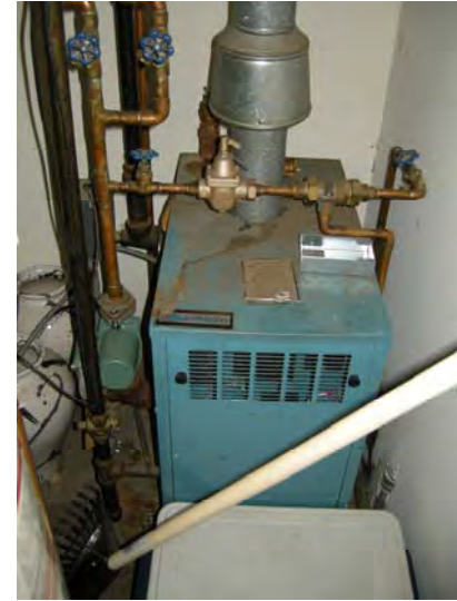
Typical gas-fired hydronic boiler
