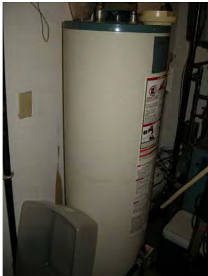
Typical gas-fired storage tank water heater
