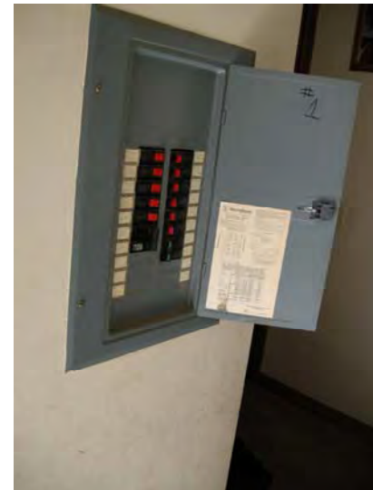
Typical unit circuit breaker panel
